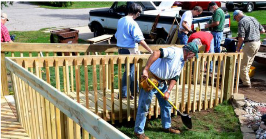
VOLUNTEERS BUILDING ACCESS RAMP
